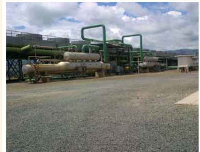
Olkaria III geothermal power project, Kenya.
