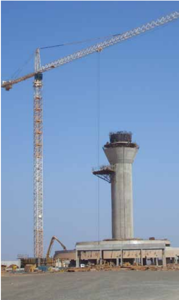
Breathing new life into Senegal's economy: work in progress on the ICF-DP supported Blaise Diagne International Airport in Dakar, Senegal.
