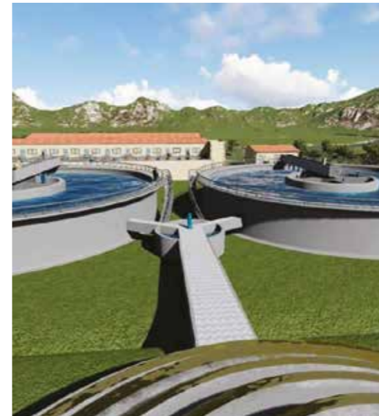
A digital representation of the Kigali Bulk Water plant in Rwanda
