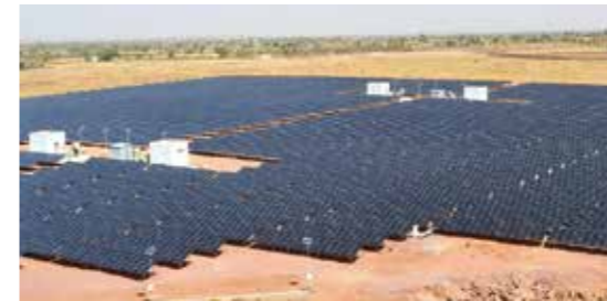
A digital representation of the Akuo Kita solar power plant, currently under construction in Mali
