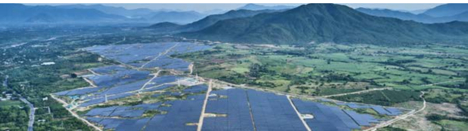
Ninh Thuan Solar Power Project
